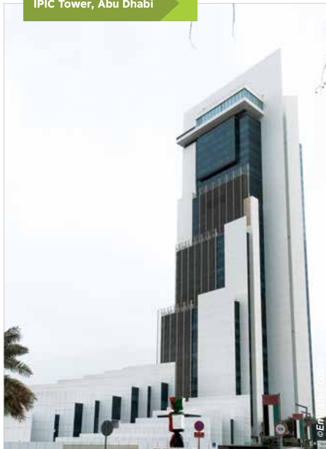
IPIC Tower, Abu Dhabi
