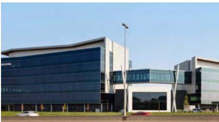
Carson Group Headquarters
